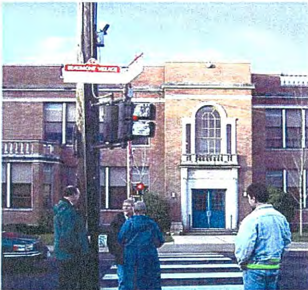
APS mounted over 12 feet high on the pole broadcast speech messages at this location in Portland. City engineers expressed concerns about intelligibility of the message.
