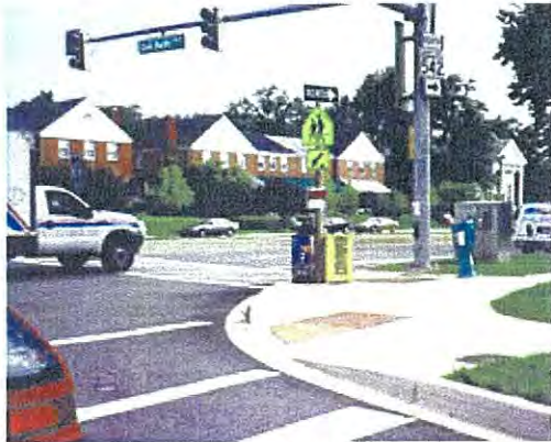
APS installed on signal pole beside crosswalk waiting location.
