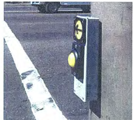
Vibrawalk pushbutton installed in Portland includes a locator tone. The arrow vibrates during the WALK interval and walk indication is provided from pushbutton or speaker mounted on the pedhead.
