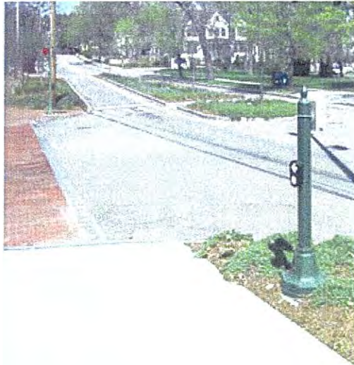
Panich APS on stub pole in Newton, Mass. arrow oriented parallel to crosswalk.
