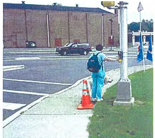
APS mounted on signal pole for crossing signalized right turn lane. A pedestrian who is blind is waiting with her hand on the pushbutton for the vibrotactile Walk indication. After the Walk indication begins, she must turn, and cross the sidewalk before beginning to cross the street.
