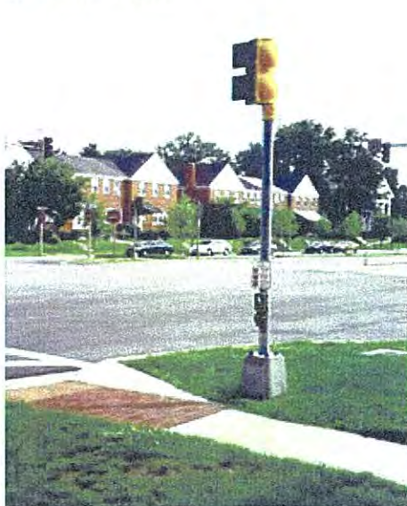
APS installed on pedestrian signal pole.
