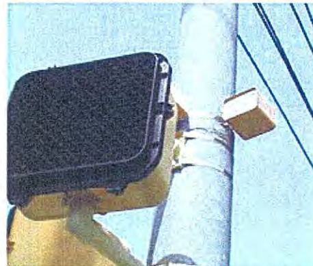
Pedhead-mounted speaker mounted on the pole as typically installed in Atlanta.
