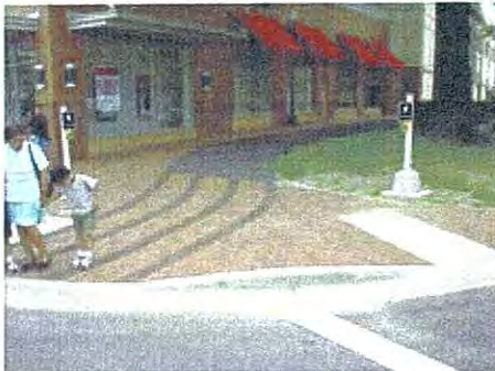
Pushbutton-integrated APS located on a stub pole beside the level landing of the curb ramp.
