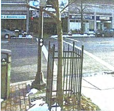
Panich APS at mid-block crossing, Newton, Mass. APS should have been mounted on side of pole closest to crosswalk, with arrow parallel to crosswalk rather than pointing up.
