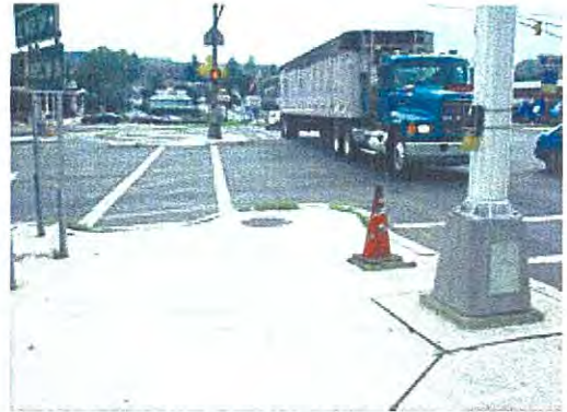
Installation of two pushbuttons on a single pole (only a single pushbutton is visible in the photo). While the pushbutton is in line with the crosswalk, the pedestrian must travel over 10 feet before reaching the street and the beginning of the crosswalk.
