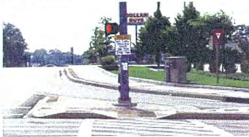
Two APS are mounted on the existing pole on this island.
