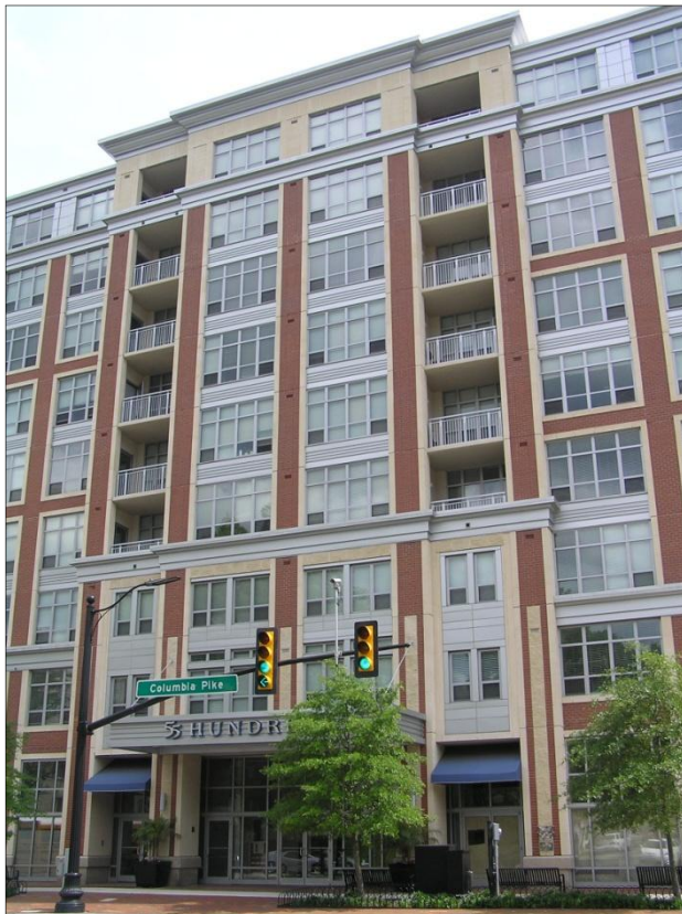
Figure 2-4. The 55 Hundred Complex on Columbia Pike
