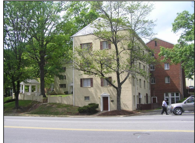
Figure 2-7. Greenbrier Apartments on Columbia Pike in Arlington
