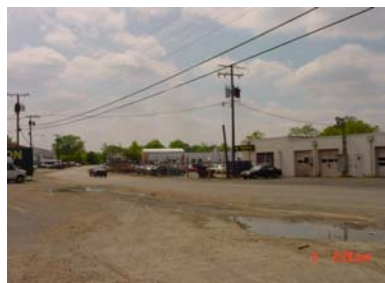
Lack of sidewalks, Center Lane
