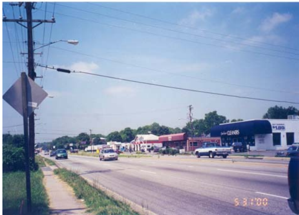
Columbia Pike Before Streetscape Project
