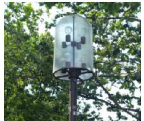
Figure 29- Pedestrian-scale light fixture
