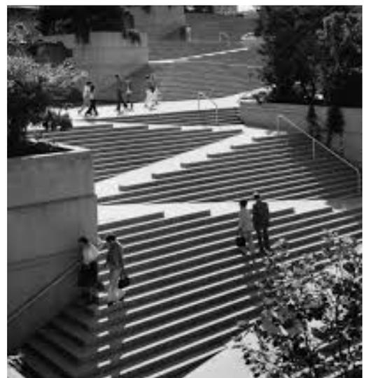
Figure 37- Integrated ramp and stair
