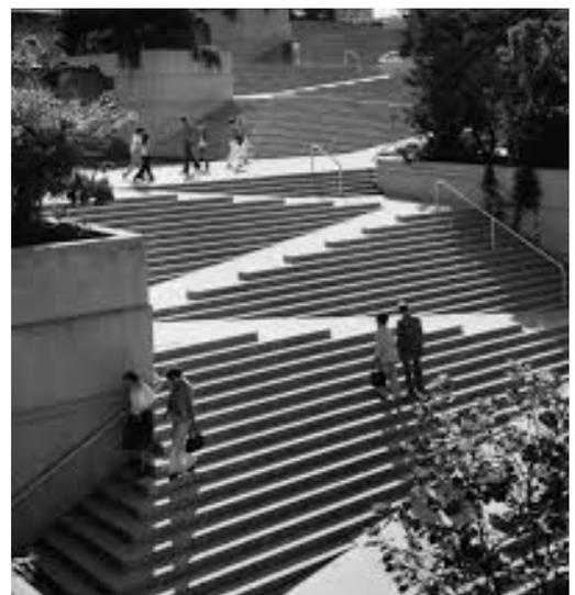
Figure 37- Integrated ramp and stair
