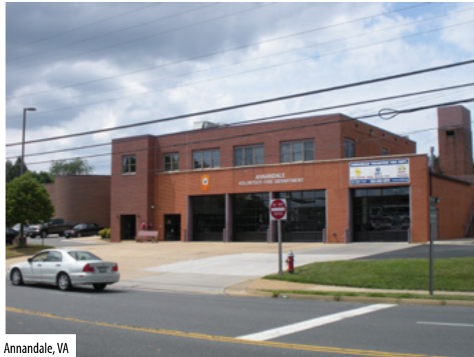
LEFT Existing Annandale Volunteer Fire Station in Annandale CRD Image Credit: Fairfax County
