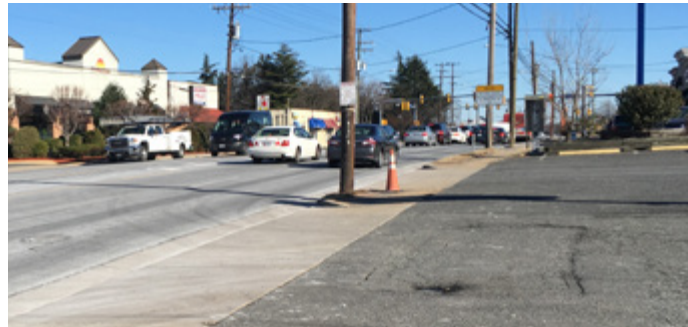
TOP Existing conditions for constrained portion of Little River Turnpike (Boulevard) in Annandale Image Credit: Fairfax County
