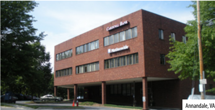
TOP Existing commercial space in Annandale CRD Image Credit: Fairfax County
