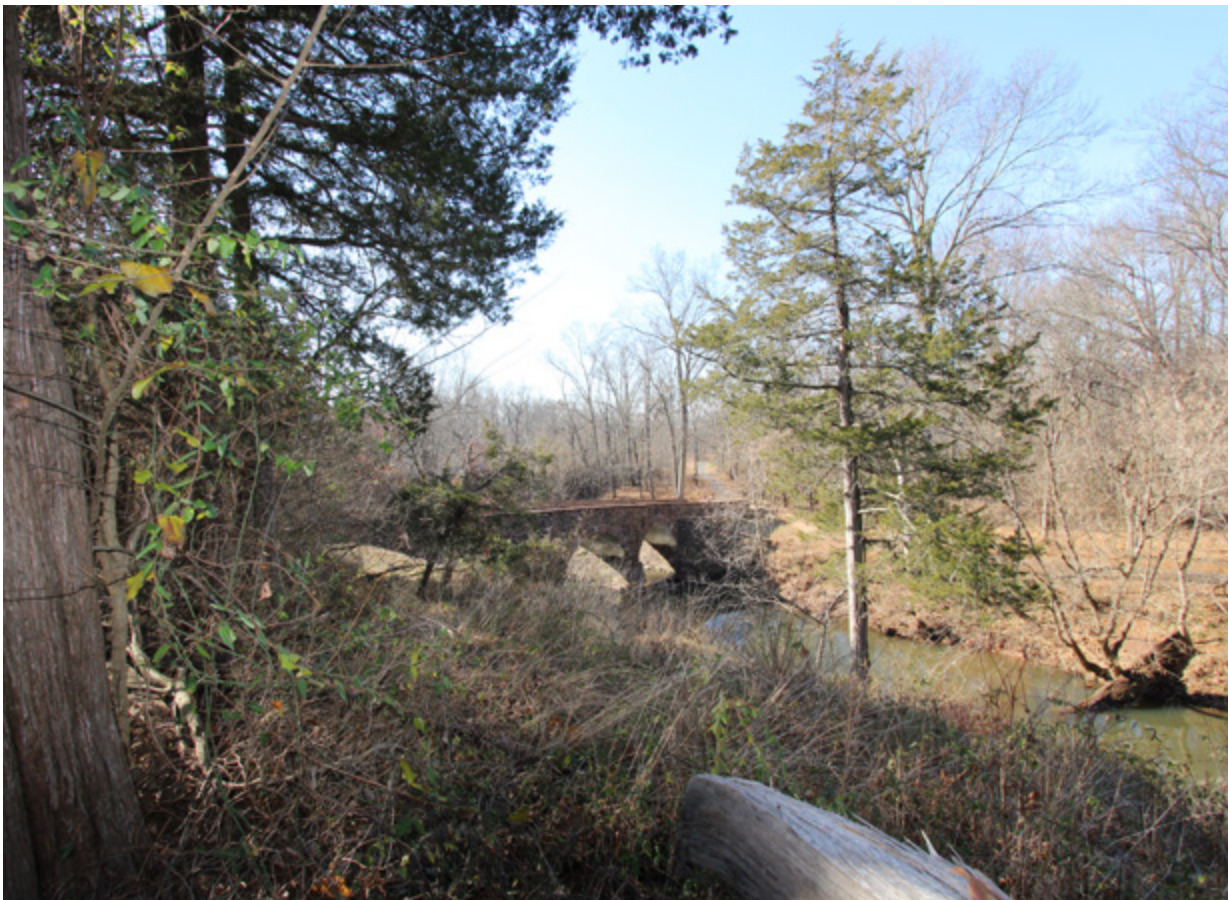
Bull Run Stone Bridge and surroundings, looking south.
