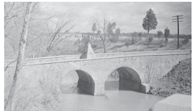
1936 view of the historic stone bridge following realignment of Route 29 National Park Service.
