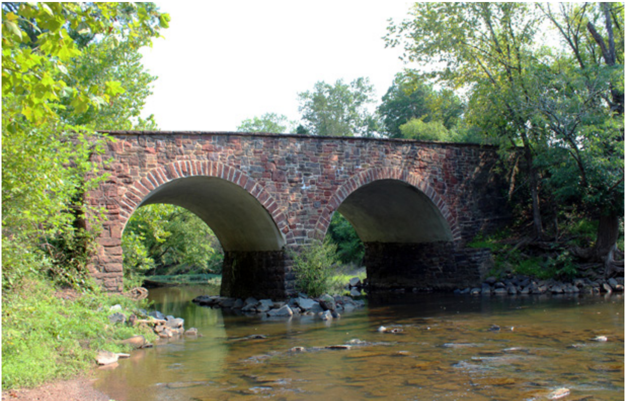
Bull Run and the Stone Bridge looking northeast.
