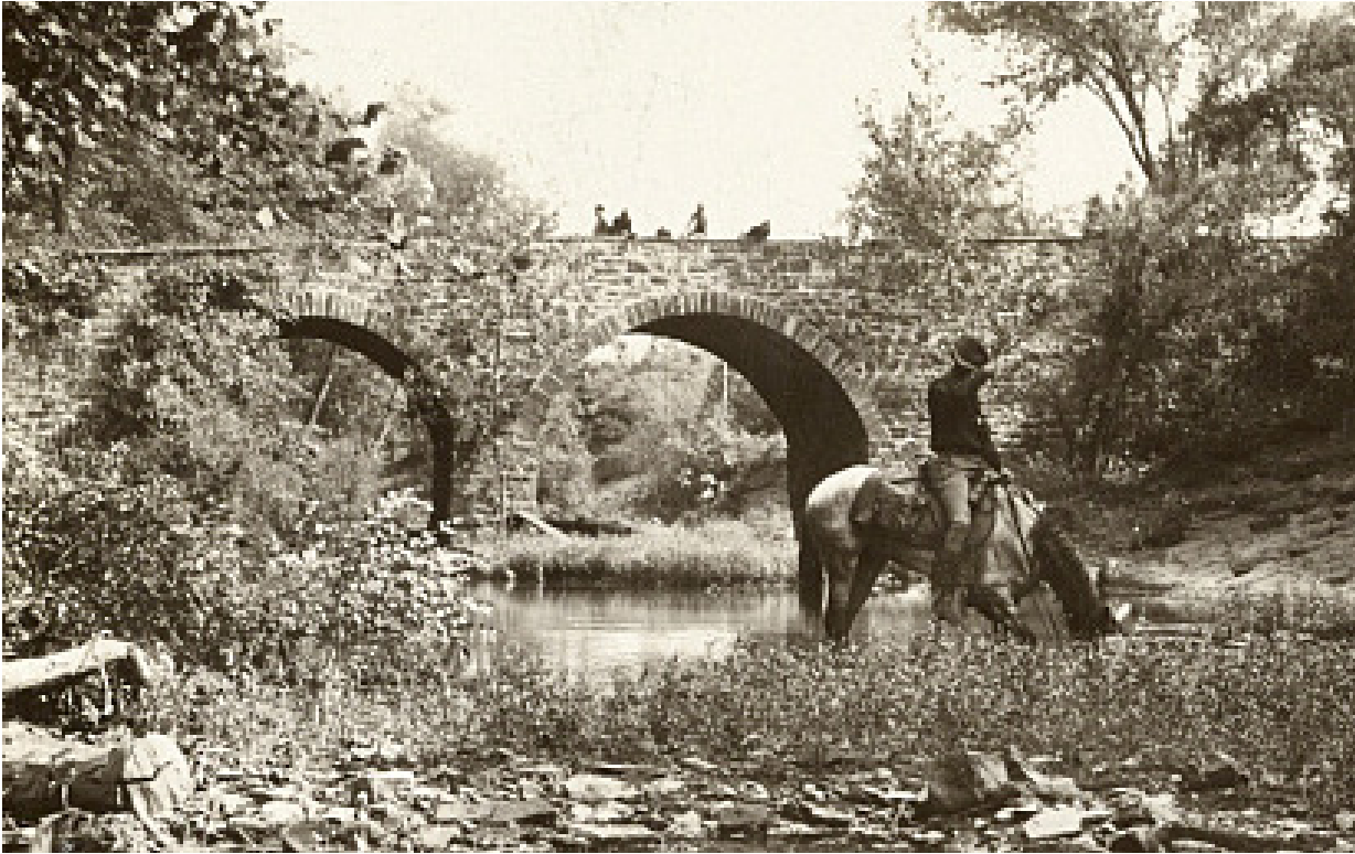
View of the historic Stone Bridge in 1923. Library of Congress
