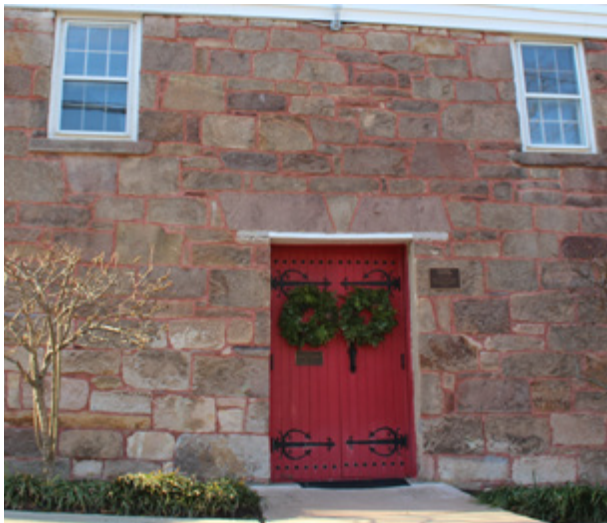
Stone construction and symmetrical fenestration pattern of Old Stone Church.
