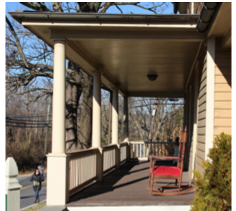
Retain original features, such as porches (recommended).
