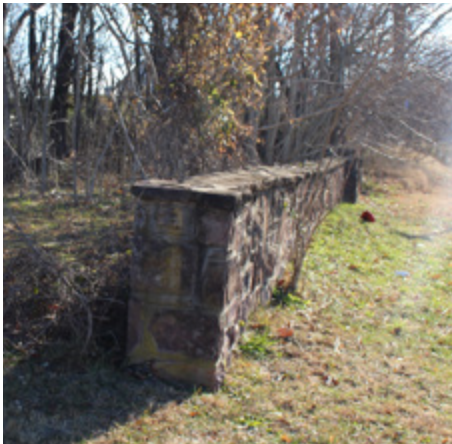
Protect existing stone walls (recommended).
