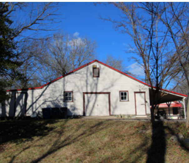
Dairy barn/shed, looking northwest.
