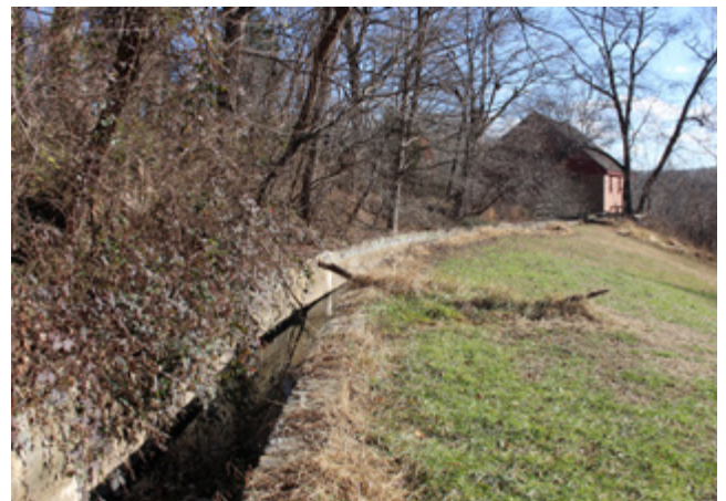
The trail race leading up to Colvin Mill to power its water wheel, looking southeast.
