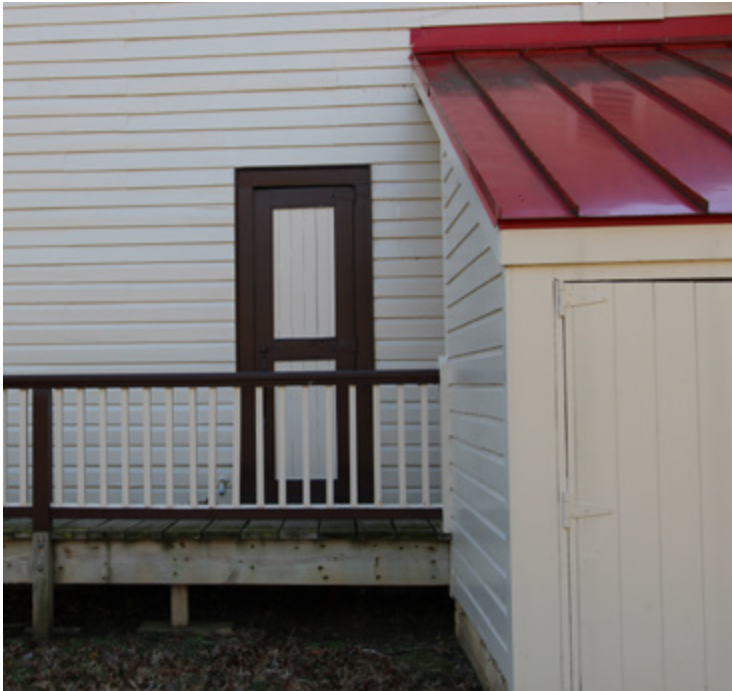
Exterior detail of the dairy barn/shed showing the German Novelty wood cladding and metal roofing.
