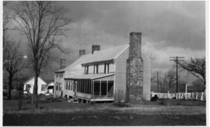
Dranesville Tavern as it appeared in 1968. Historic American Buildings Survey (HABS).
