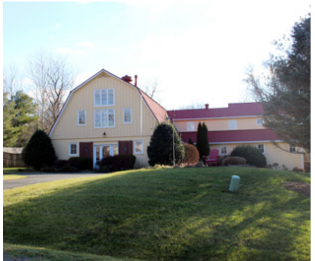
McDannald Barn and Outbuildings
