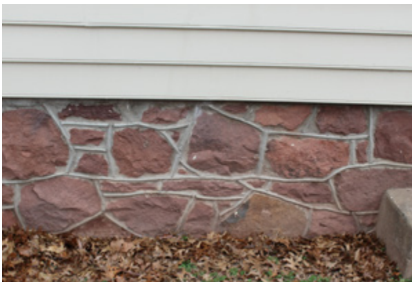
Detail of the tavern's sandstone foundations and beaded weatherboard siding.
