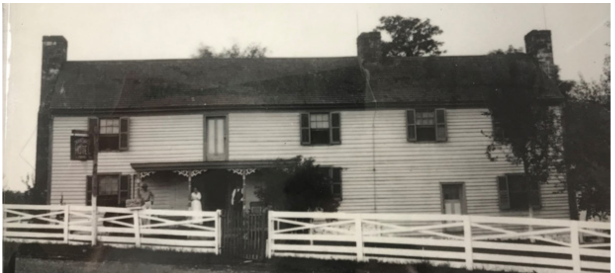
Dranesville Tavern in 1918. Fairfax County Public Library Virginia Room.
