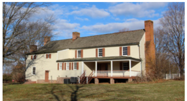
Dranesville Tavern as it appears today, looking north.
