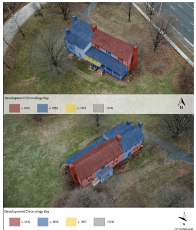
Two aerial schematics showing the building chronology of Dranesville Tavern. EHT Traceries .
