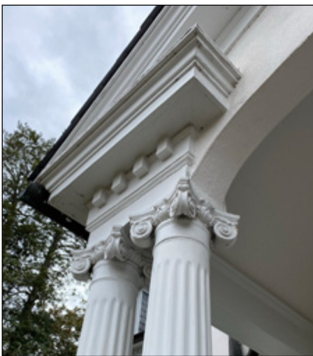
Ionic columns and dentil molding, Wellington at River Farm HOD.
