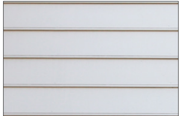
Beaded weatherboard siding at the Dranesville Tavern HOD.
