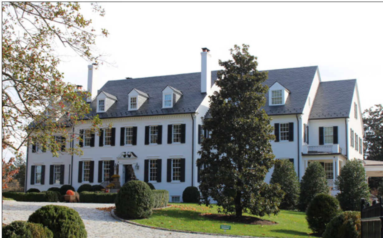
Hickory Hill, a historic property in the Langley Fork HOD.
