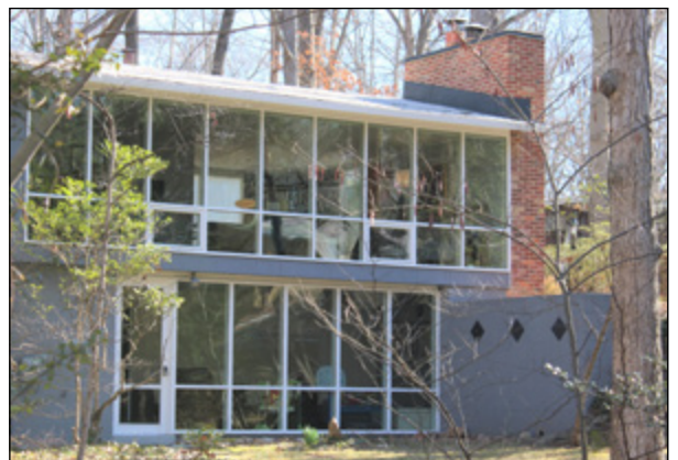
Building in the Hollin Hills HOD with a high proportion of windows resulting in a low solid-to-void ratio.
