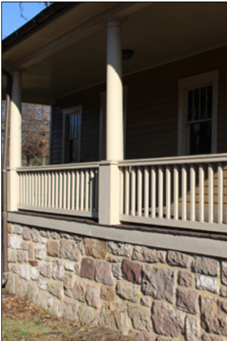
Stone foundation in the Centreville HOD.
