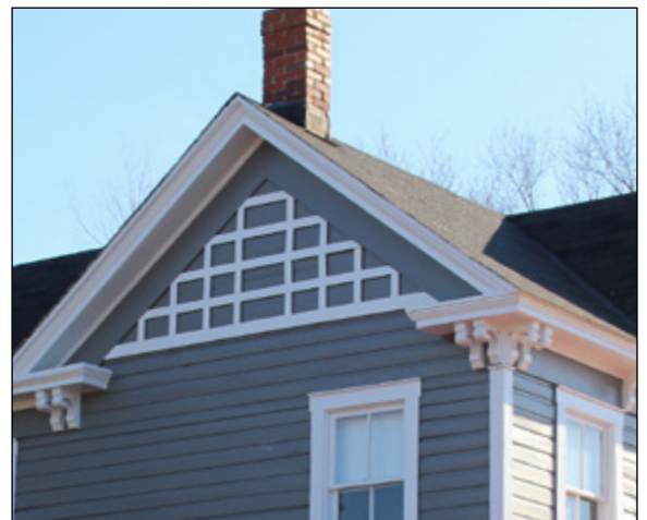
Cornice brackets and applied decorative stickwork in the Centreville HOD.
