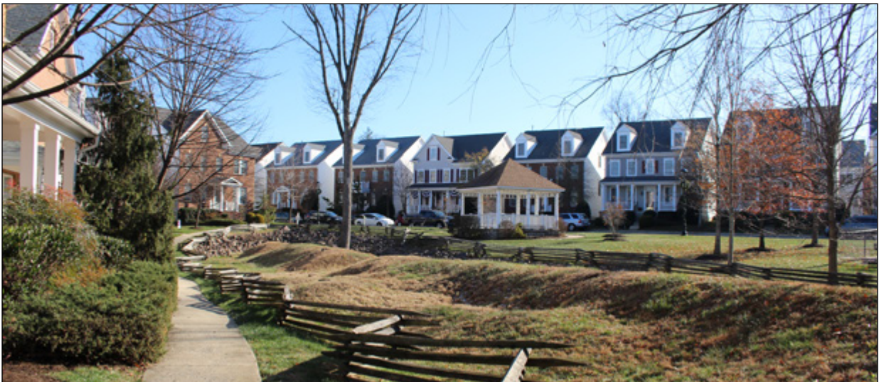
New construction within the Centreville HOD.
