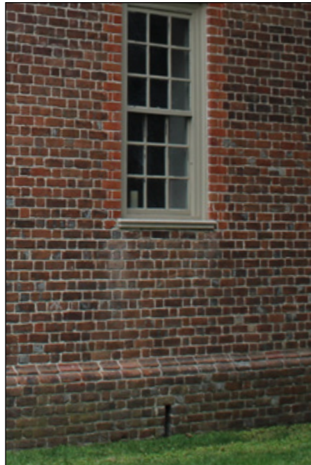
Brick foundation at the Pohick Church.
