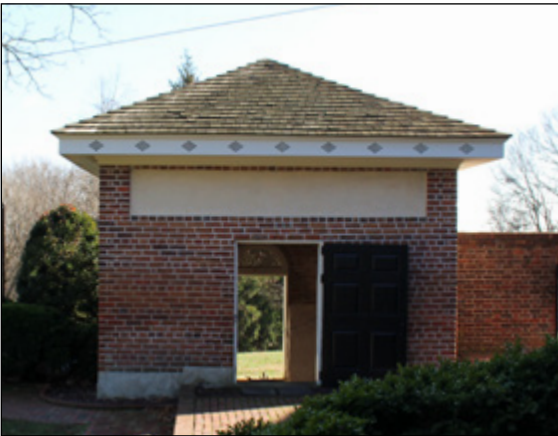
Pyramidal-hipped roof covered in wooden shingles in the Woodlawn HOD.
