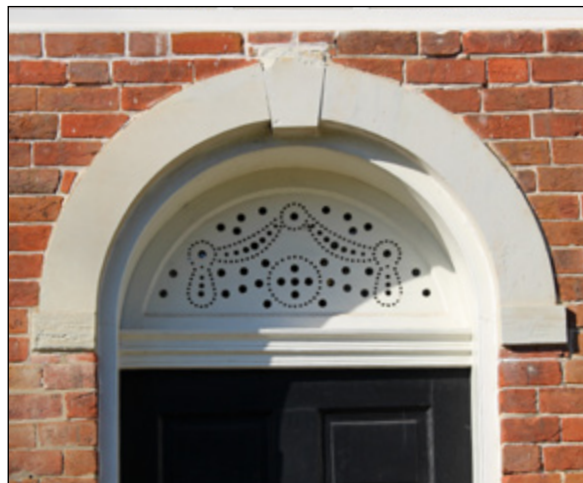
Blind transom with decorative wood panel and keystone arch in the Woodlawn-Pope Leighey HOD
