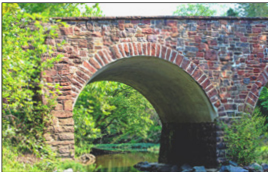
The restored Bull Run Stone Bridge.
