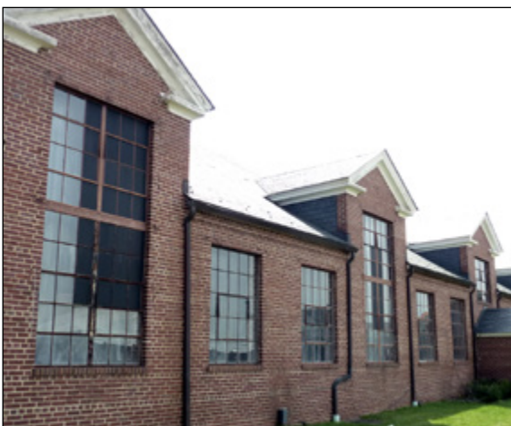
Steel-sash windows at the Lorton Prison.
