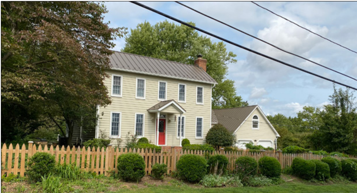
Garage addition that is subordinate to the historic building.
