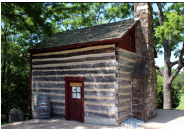
Building in the Sully HOD with a single door opening resulting in a high solid-to-void ratio.
