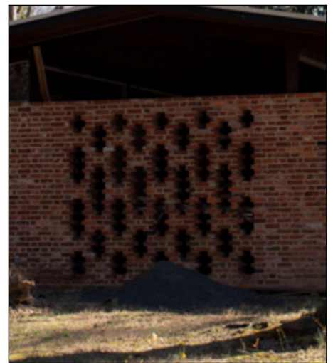
Decorative brick screen wall, Hollin Hills HOD.
