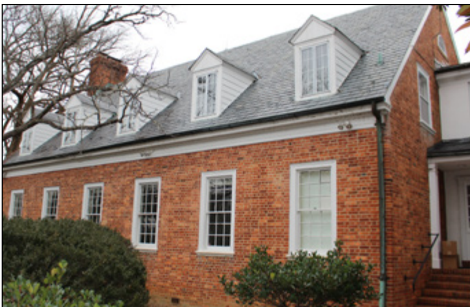
Double-hung windows and paired casement windows on a building in the Wellington at River Farm HOD.
