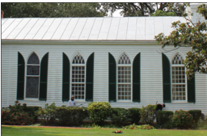
Gothic arch windows at the St. Mary's Church.
