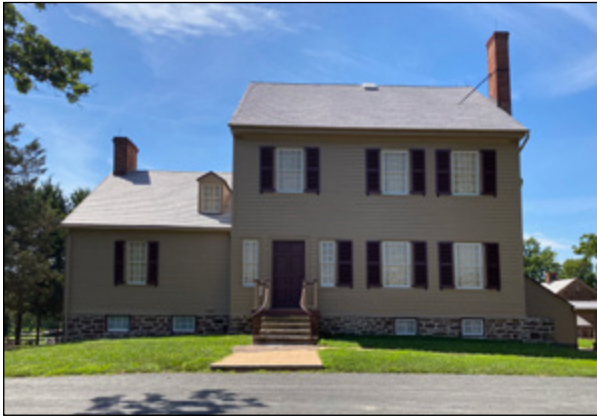
Main historic building volume and secondary wing on Sully.
