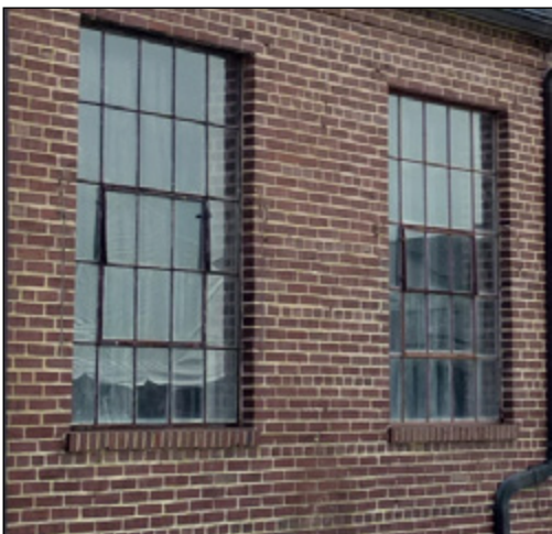
Brick wall cladding laid in an American bond at Lorton Prison.
