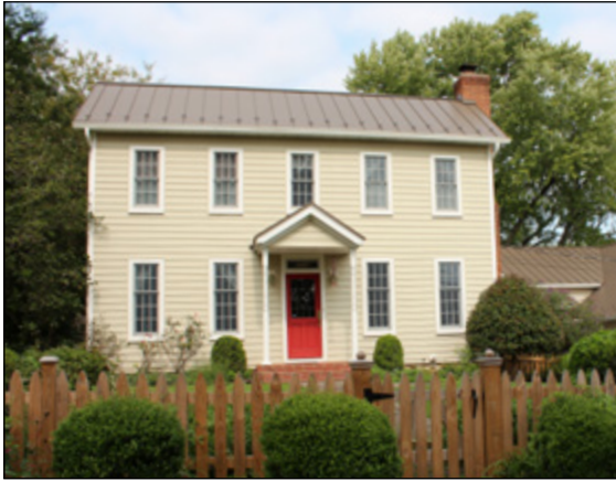
Side-gabled roof covered in standing seam metal in the St. Mary's Church HOD.
