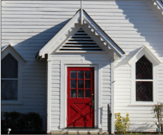
Single-leaf partially-glazed wood door in the Centreville HOD.
