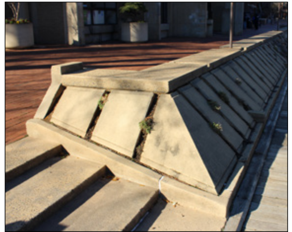
Grooved concrete site wall in the Lake Anne HOD.
