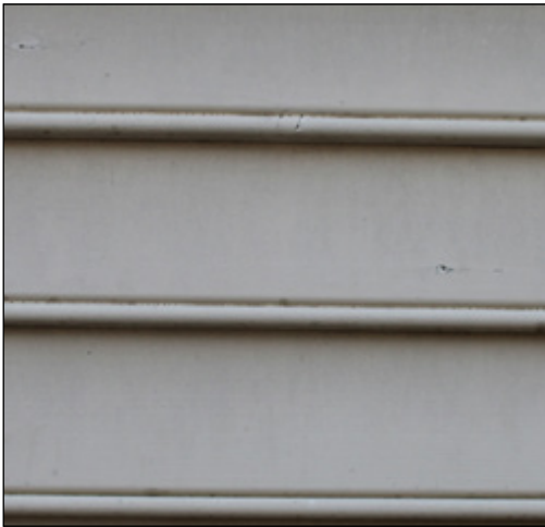
Beaded clapboard siding at Huntley.
