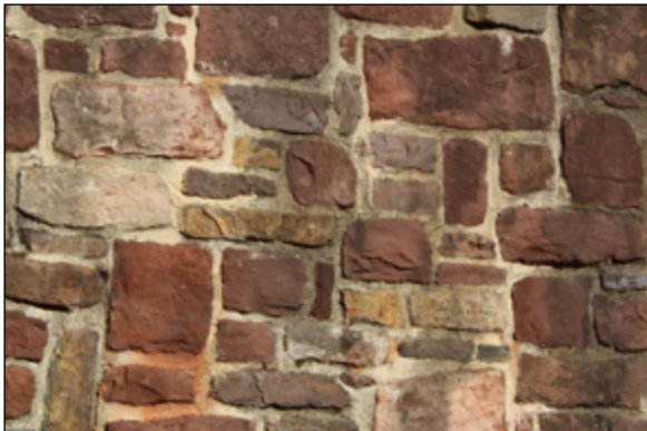
Gray and red sandstone at the Bull Run Stone Bridge HOD.
