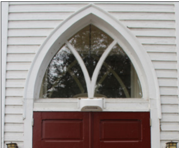
Gothic Revival-style transom window above a paneled wood door in the Langley Fork HOD.
