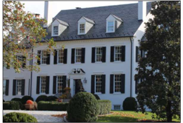
House in Langley Fork with hierarchy of windows that reduce in size at upper floor levels.
