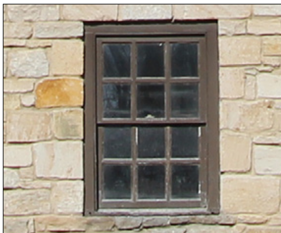
Double-hung wood-sash window in the Woodlawn HOD.
