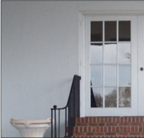
Stucco coating on walls on Wellington at River Farm.
