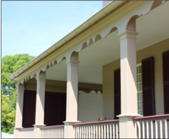
A porch with ornamental trim in the Sully HOD.
