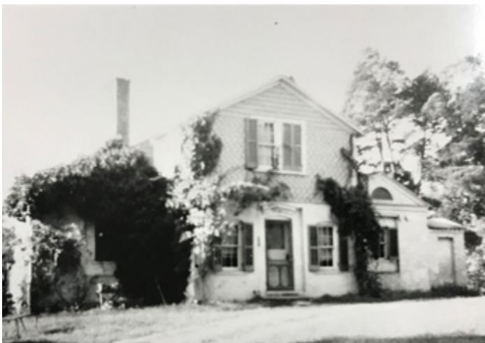
Undated photograph of Huntley’s north elevation. Fairfax County Public Library, Virginia Room.
