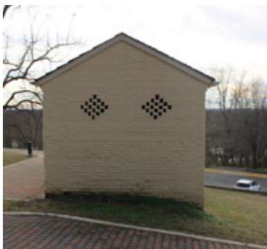
Building foundation and necessary.
