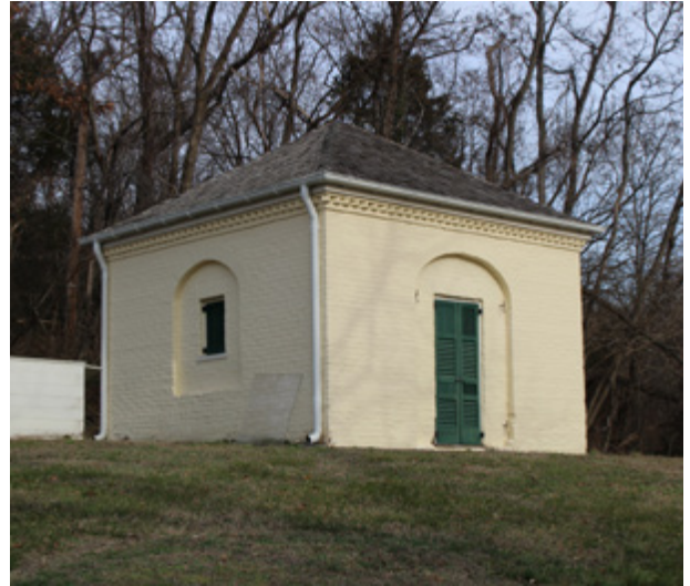
Root cellar. View looking northeast.
