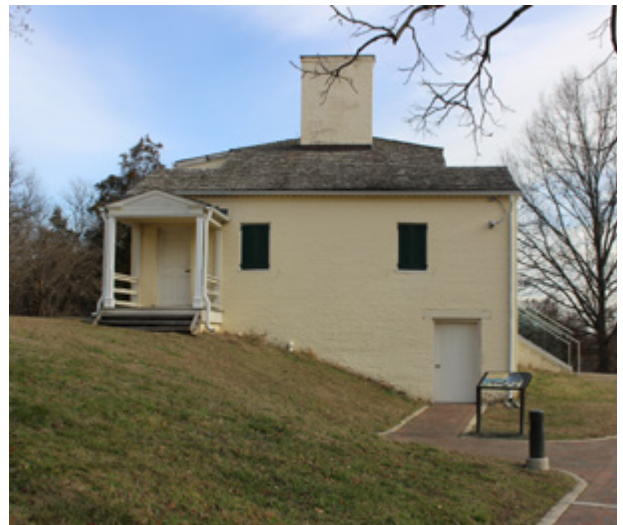
West elevation of Huntley; view looking east.
