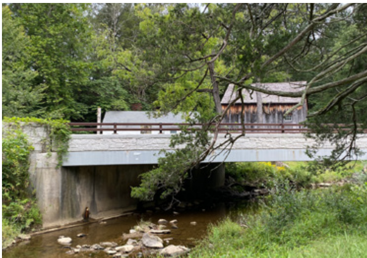
Pope's Head Road bridge crossing Piney Branch.
