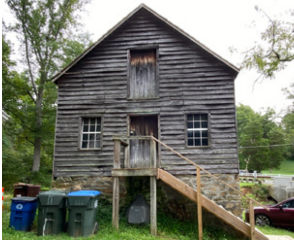
Two-and-one-half-story mill building.
