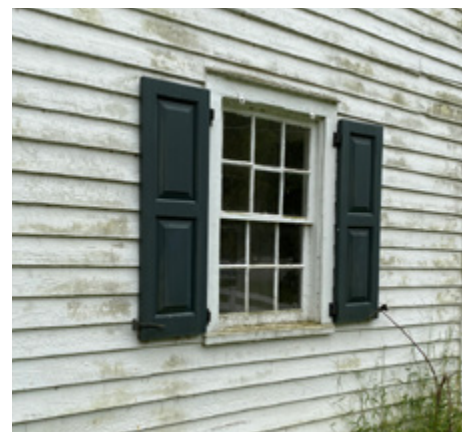
Retain architectural features including wood cladding and wood windows (recommended).
