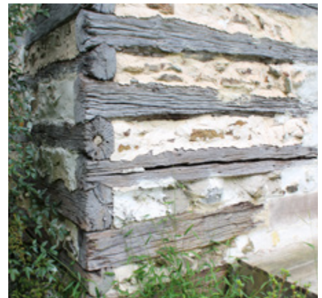
Retain original v-notched log construction (recommended).
