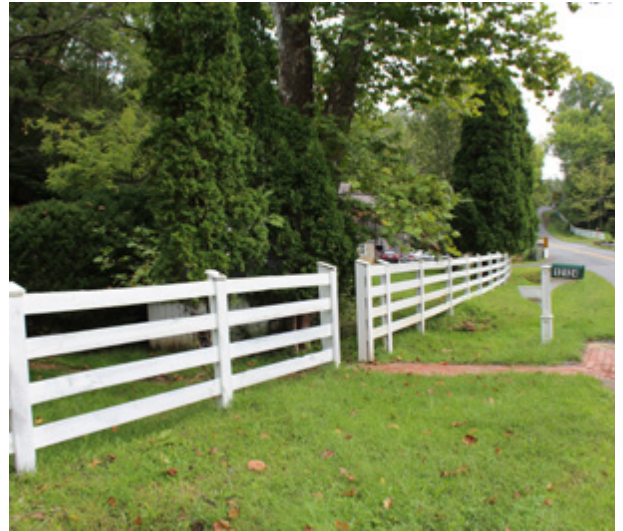
Wood board fencing along Pope's Head Road.
