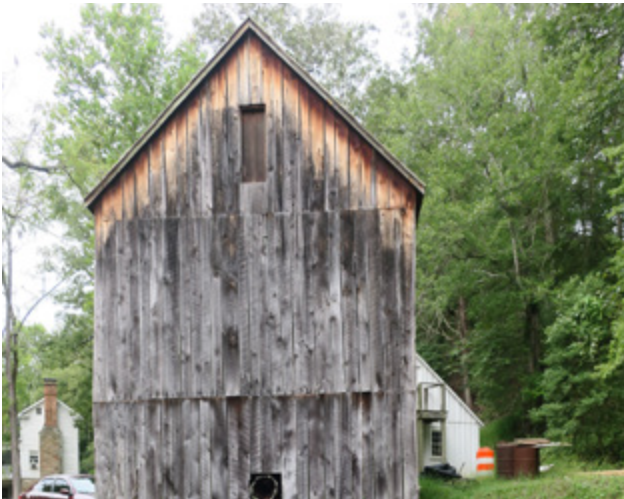
Robey's Mill, looking west, with the Miller's House at image left. The shed is partially pictured at image right.
