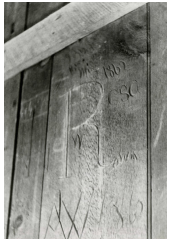
Remnant of Civil War-era carvings on the interior of the mill (1977). National Register of Historic Places Registration Form.
