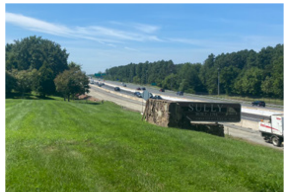
Open berm and signage along Sully Road.
