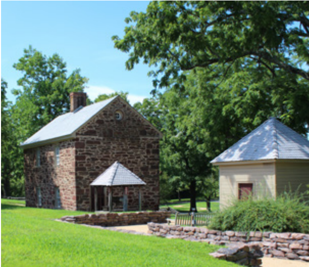
Smokehouse (historic), stone dairy (historic), and well (noncontributing), looking southwest.
