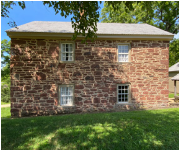
Stone dairy with regularly spaced window openings filled by double-hung wood-sash windows.
