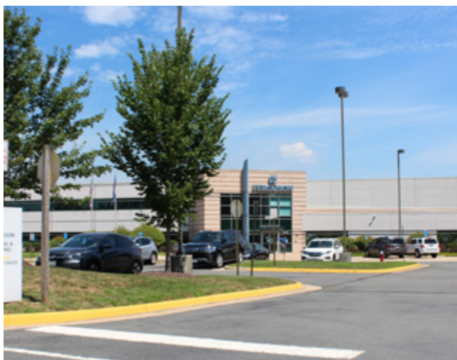
Use of design and materials that are incompatible with the HOD (not recommended).
