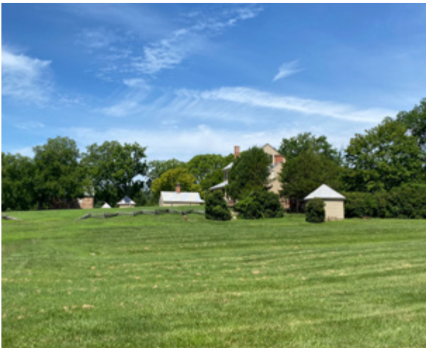
View west toward Sully house and outbuildings (office at left).
