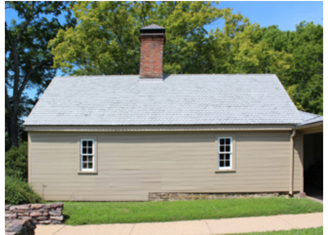
Kitchen house, looking west.
