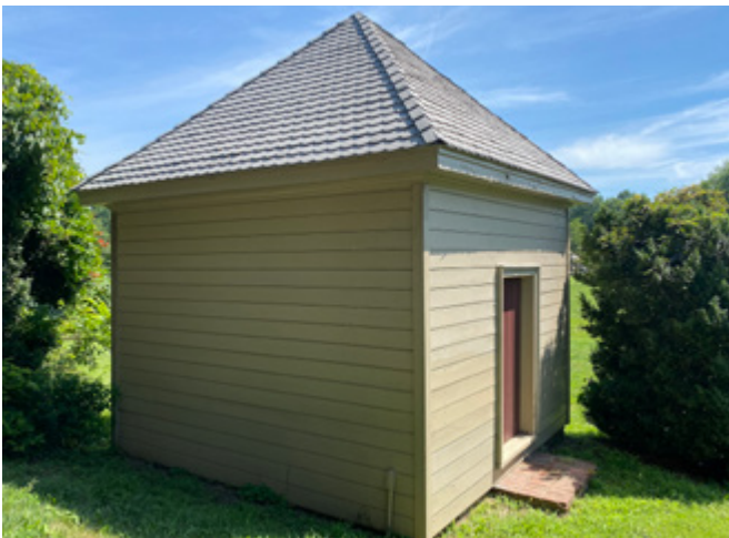
Office, looking northeast.
