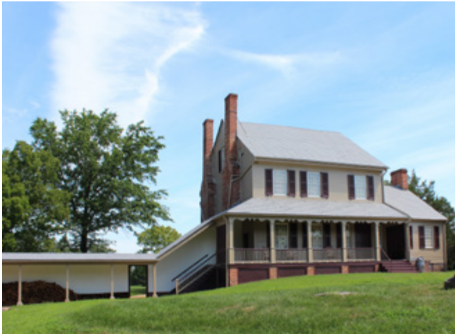
Sully house and covered walkway, looking north.
