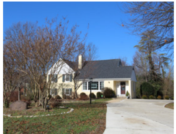
Low scale construction with adequate screening that does not impact views toward Woodlawn or the Pope-Leighey House and other historic resources (recommended).
