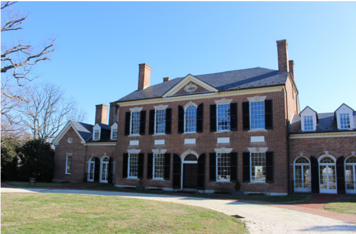
Woodlawn's north elevation; view looking southeast.
