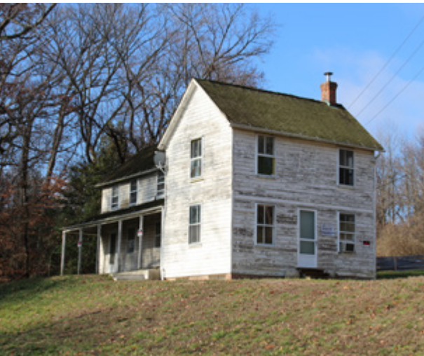
East and south elevations of the Otis T. Mason House.
