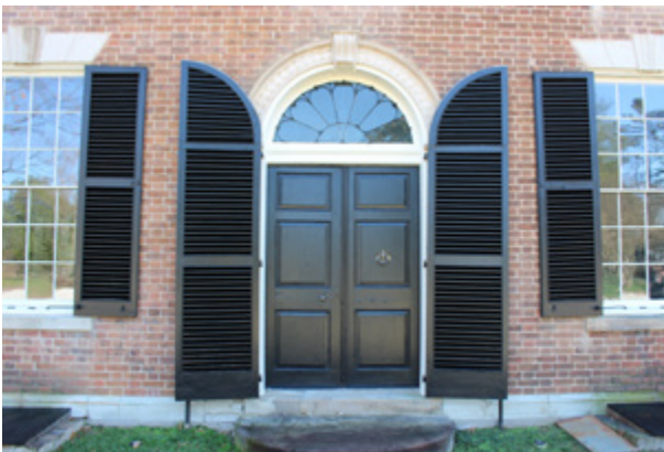
Detail of the main entrance on the north elevation.
