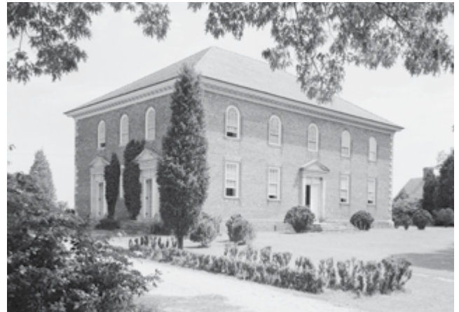
Pohick Church as it appeared in the 1930s. Historic American Buildings Survey (HABS) .
