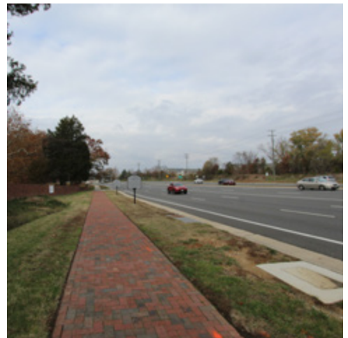
Encroaching upon the Pohick Church property for road widening (not recommended)
