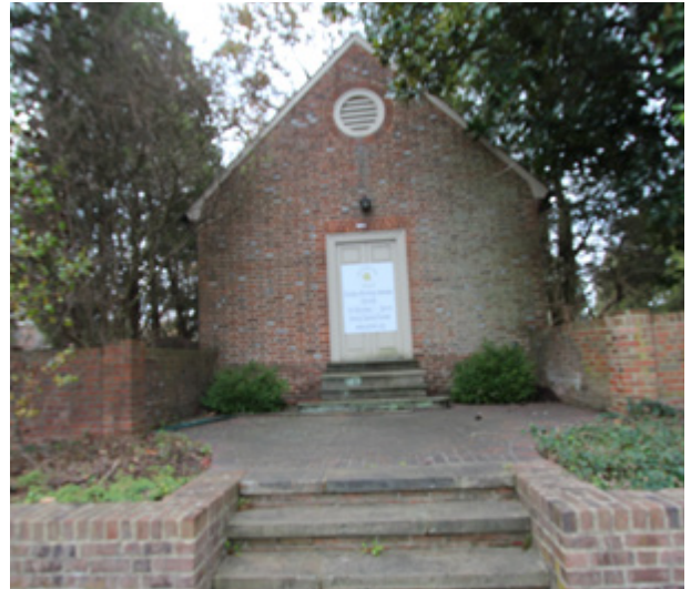
Vestry house, looking south from Route 1.
