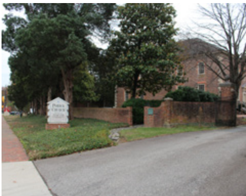
Preserve brick site walls and continue brick paving where necessary (recommended)
