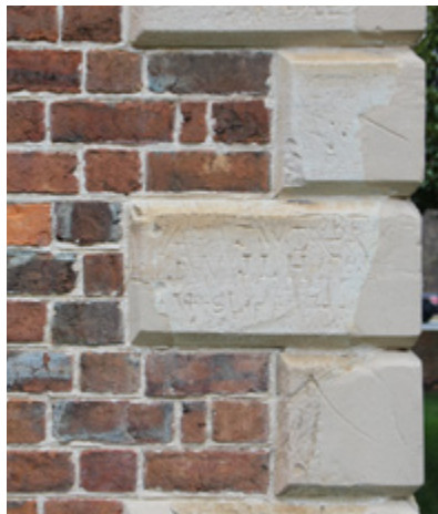
Use of materials, design features, and color palettes that are compatible with the church complex (recommended)
